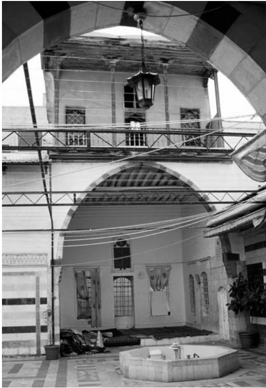
Figure 3.1 A view of the internal courtyard of ‘Abd al-Ghani’s house after several renovations. The room above the arched space is his room, which is rendered directly inaccessible (author).
