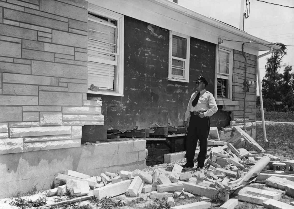
A policeman inspects damage after the Wades' house was dynamited.
